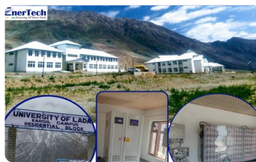
Application: Education University Rating: 100kW/200kWh Site location: Ladakh, India
