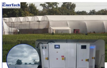
Application: Poly House Rating: 200kW/200kWh Site location: Nashik, India
